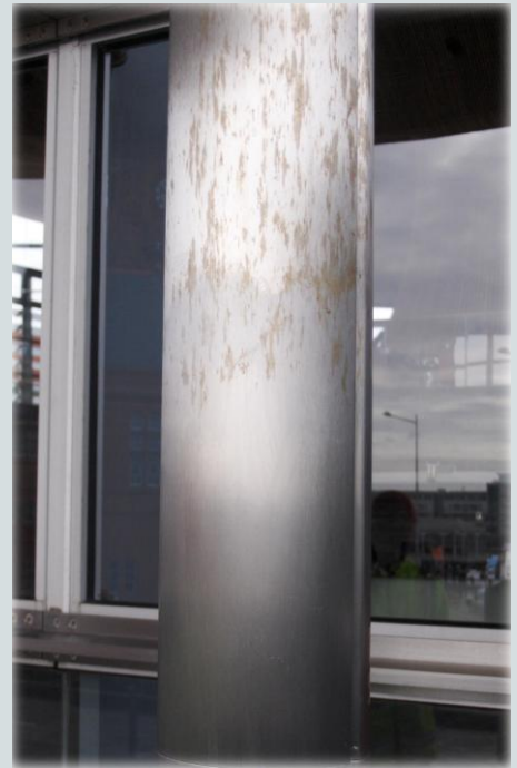
This column showed signs of corrosion shortly after installation. The lower area has been treated with Cleaner 160.
